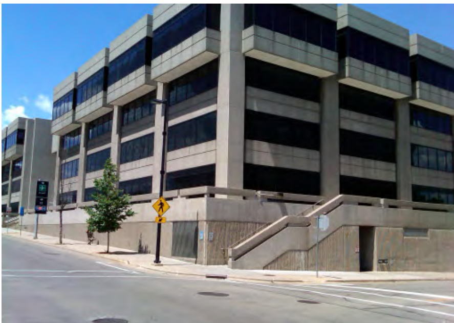
DWD is headquartered at the GEF 1 State Office Building in Madison, Wisconsin.
