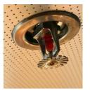
When the air temperature above the fire rises to a certain temperature, a fire sprinkler system is activated. The sprinkler sprays water forcefully over the flames, extinguishing them completely in most cases, or at least controlling the heat and limiting the toxic smoke until the fire department arrives. Only the sprinkler(s) nearest the fire activate. Smoke alone does not activate sprinklers.
